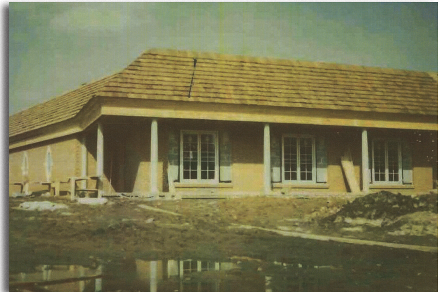
Construction of the new Swanson Chapel
