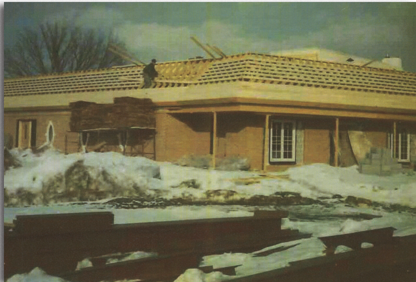
Construction of the new Swanson Chapel
