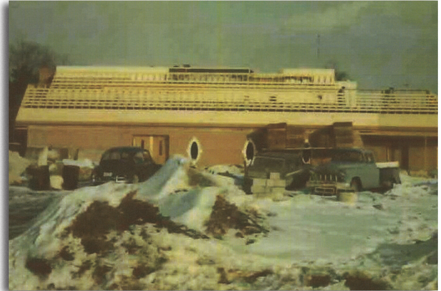
Construction of the new Swanson Chapel
